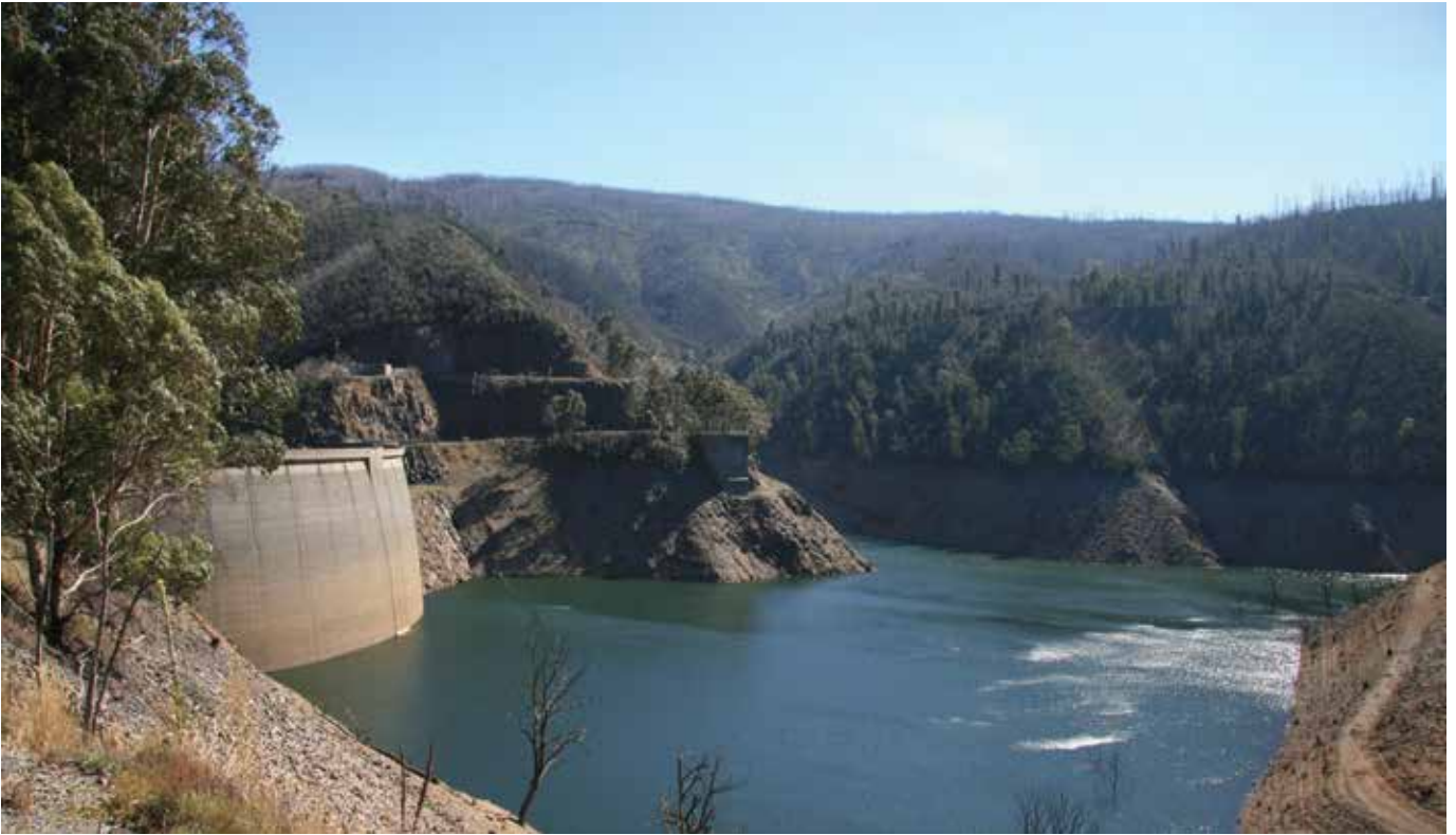
Tumut Pond Dam wall. Photo: Mick Stanic
